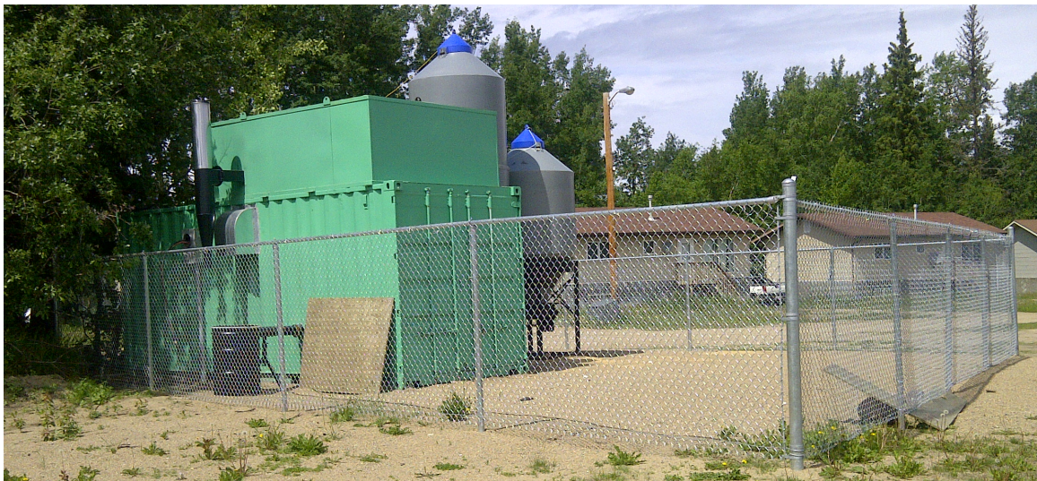
Meadow Lake Tribal Council's large boiler demonstration project in Canoe Lake, SK. It heats four teacherages. The wood pellets are stored in the grey cylinders and automatically delivered to the boiler.
